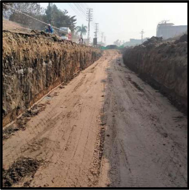
Picture 86: Sewer Bed Preparation
