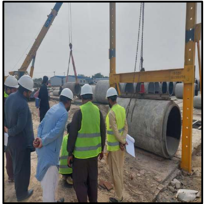
Picture 44: 03-Edge Bearing Test
