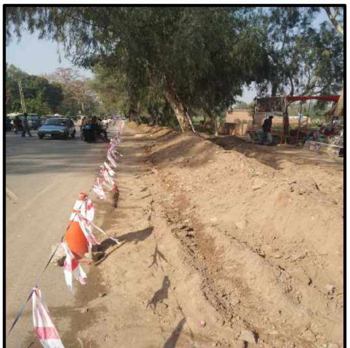
Picture 18: View of Trench After Pipe Laying
