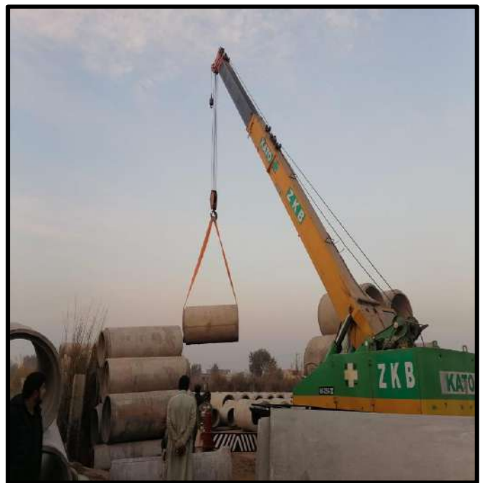
Picture 60: Hauling of Pipe in Progress
