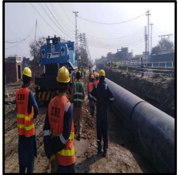
Picture 83: Backfill Restoration
