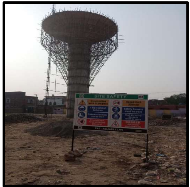
Picture 89: Construction of OHR in Progress
