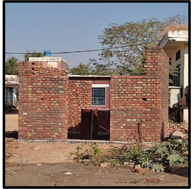
Picture 87: Brick work of Pump Room in Mayana Pura
