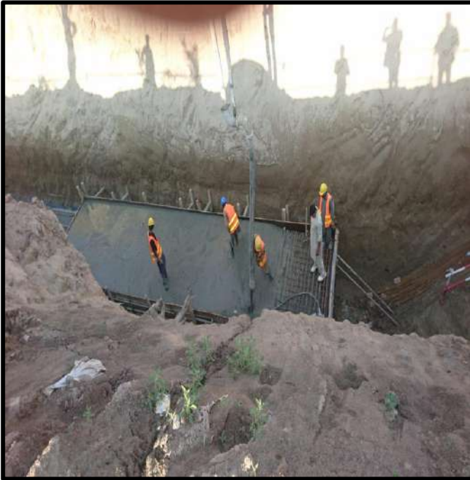
Picture 35: Concrete Roof Slab in Progress
