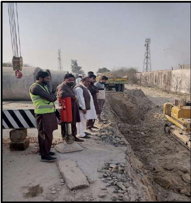
Picture 43: Sewer Bed Preparation
