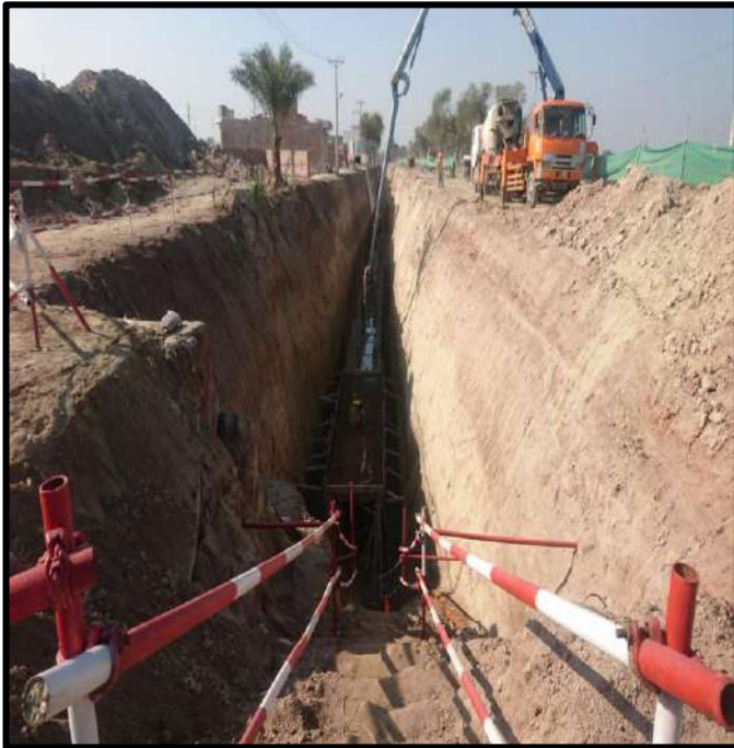
Picture 33: Acces to the Conduit which is in Progress
