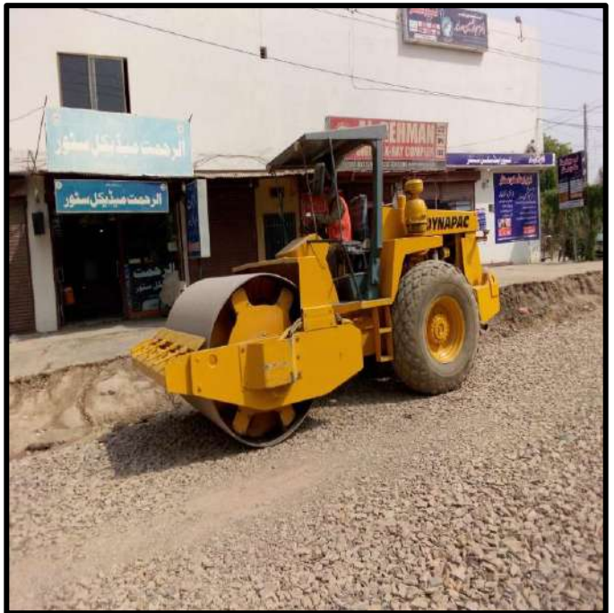
Picture 50: Compaction of WBM In Progress
