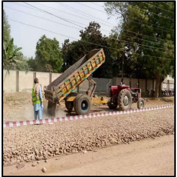
Picture 48: Water Bound Macdum at Fateh Sher Road-01
