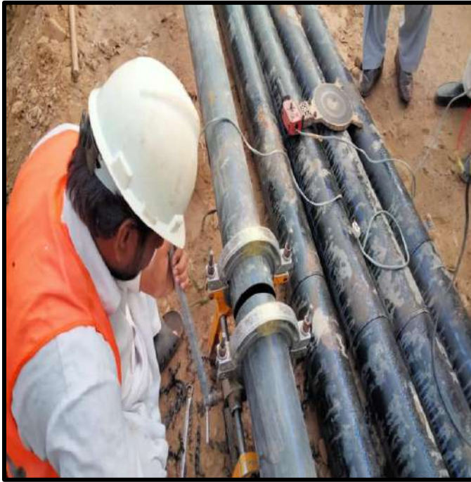
Picture 19: HDPE Pipe Welding and Jointing in Progress
