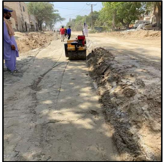
Picture 56: Compaction after sewer laying in progress
