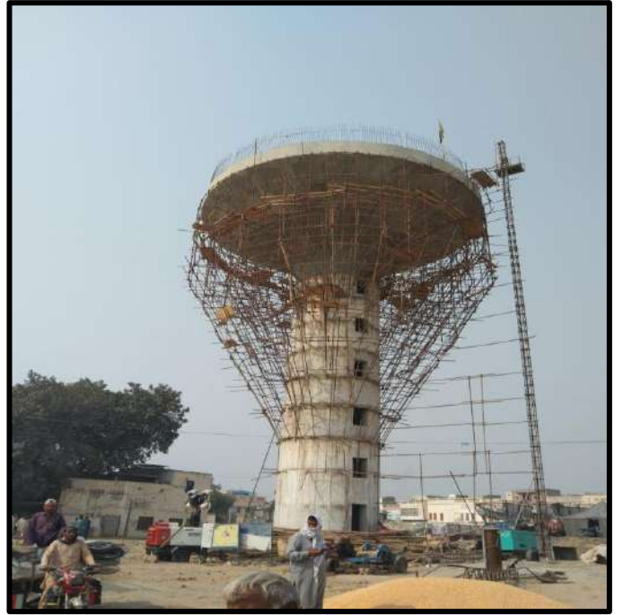
Picture 24: Removing of OHR Shuttering in Progress
