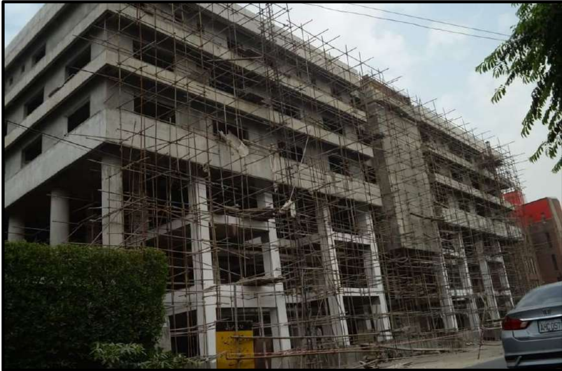
Picture 97: Front Elevation of PLGA Lahore
