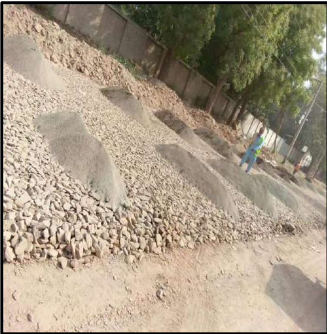
Picture 49: Laying of WBM in Progress
