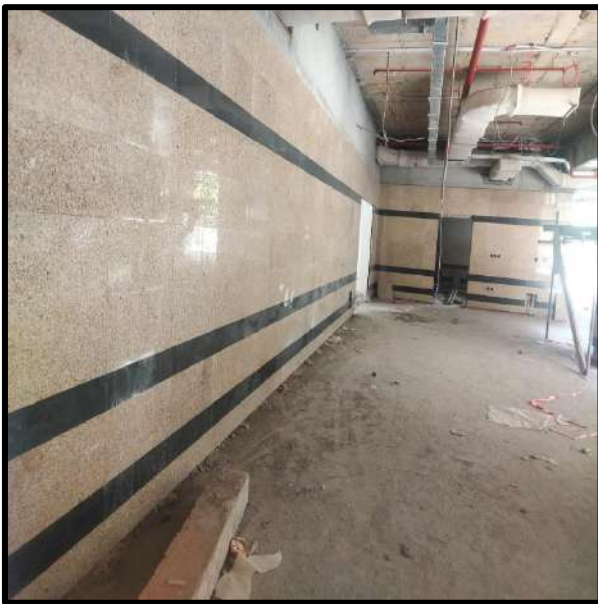
Picture 98: Fixing of Granite on Walls
