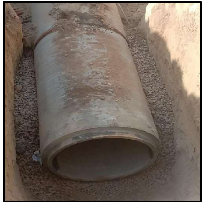
Picture 46: Sewer Laying
