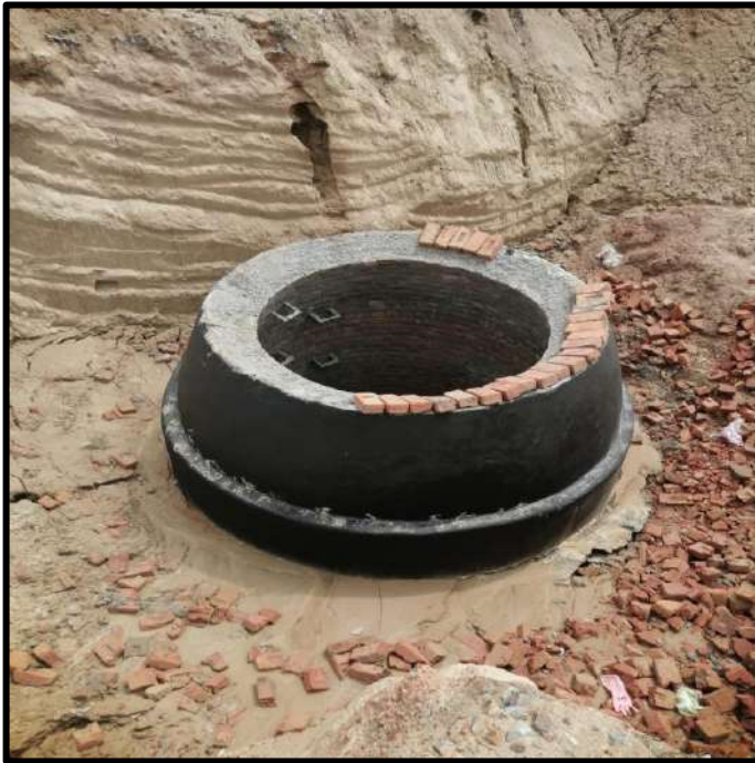
Picture 31: Manhole under Construction
