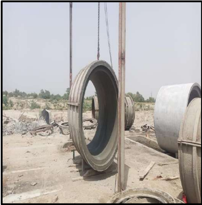
Picture 39: Laying of 48" Dia Pipe at Multan Road
