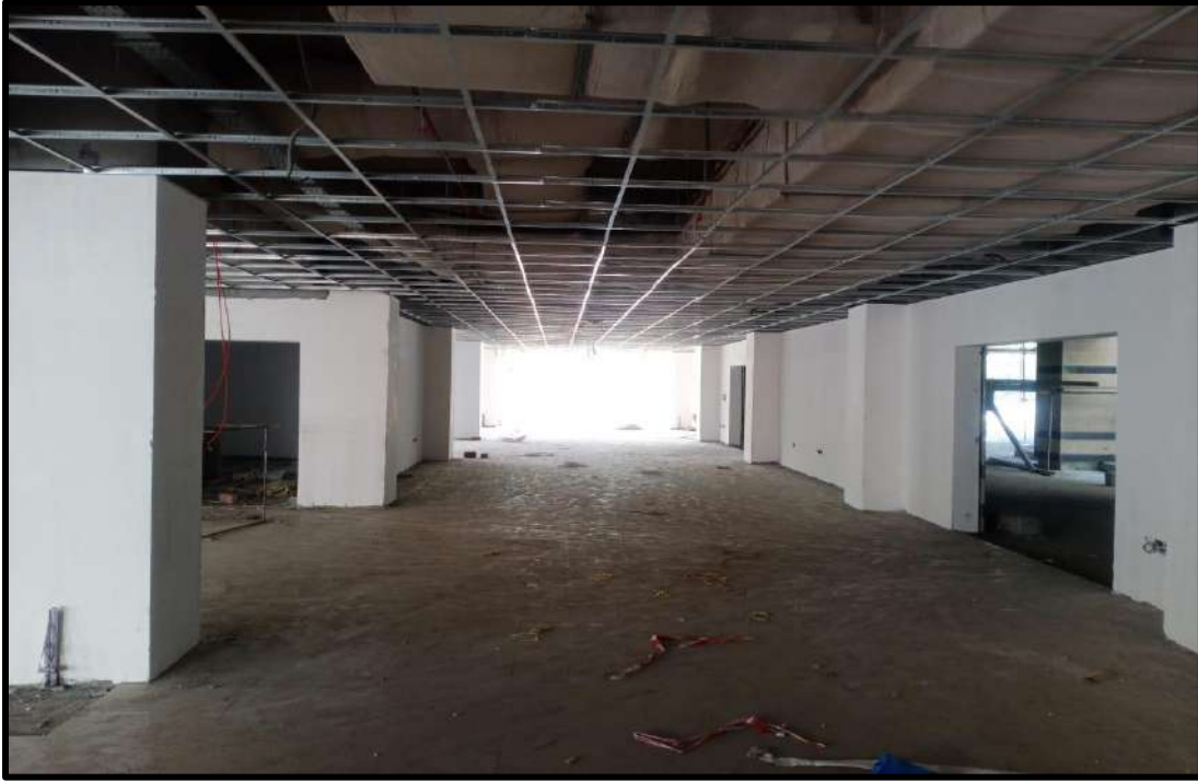
Picture 100: Paint work and fixing of Ceiling Frame
