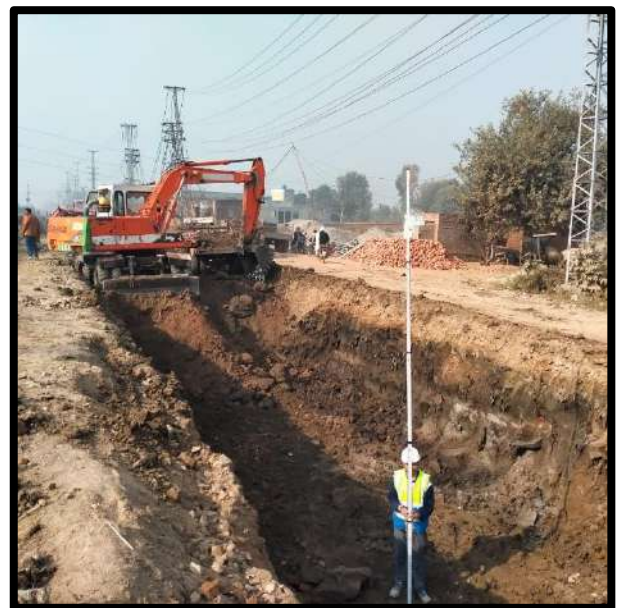
Picture 85: Bed Preparation for layinf of Forcemain
