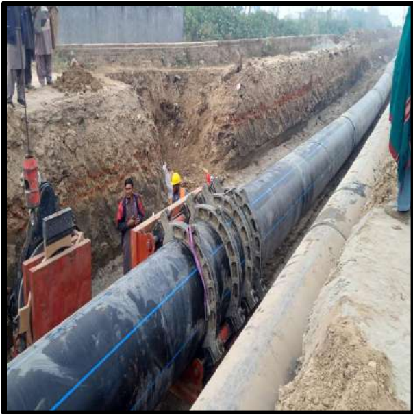
Picture 82: Conduit Placement (Night Shift)
