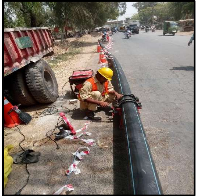
Picture 20: HDPE Pipe Jointing At UC-10
