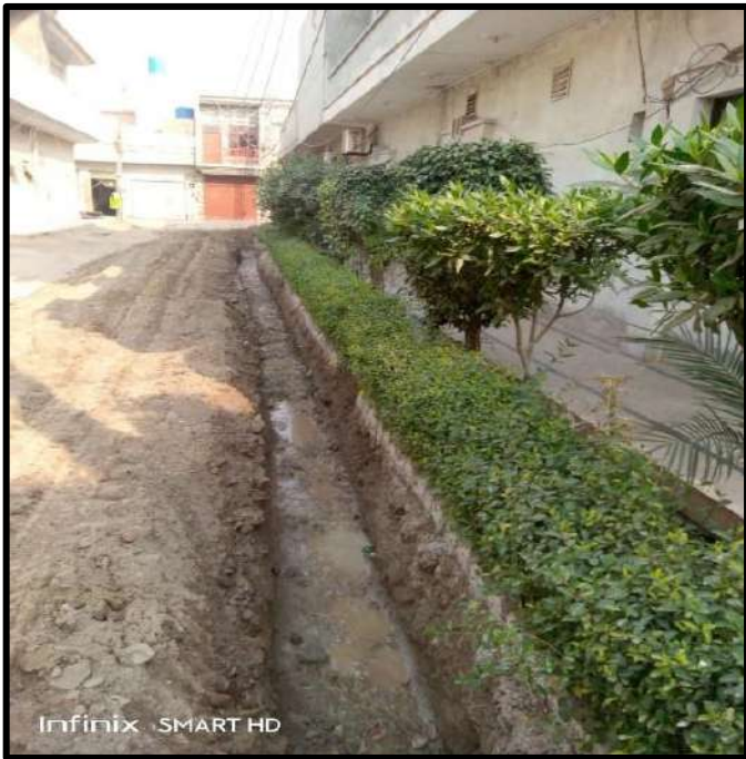
Picture 17: View of Trench After Pipe Laying
