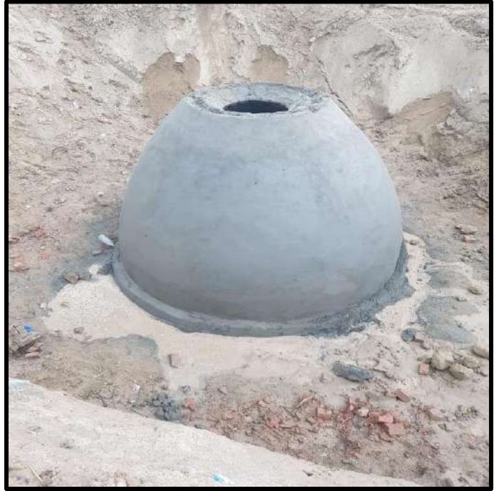
Picture 32: Manhole under Construction
