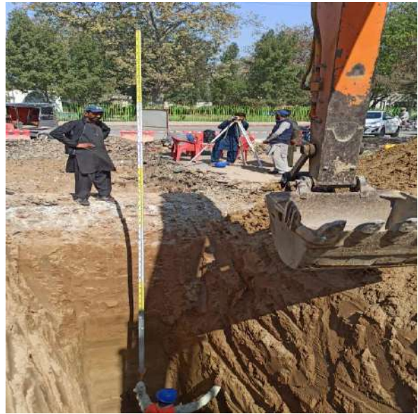
Picture 30: Excavation Work in Progress
