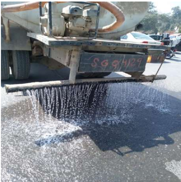
Picture 29: Water Sprinkling in Progress
