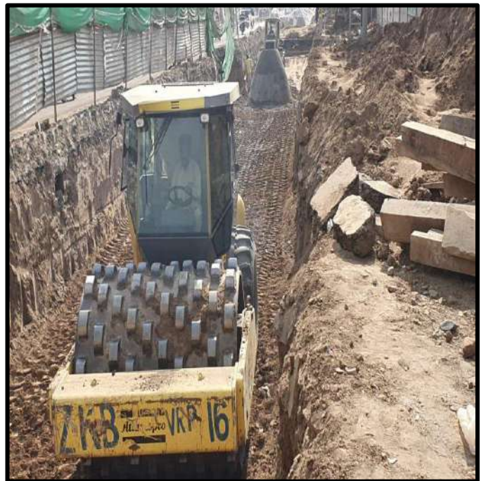
Picture 62: Compaction of Backfill
