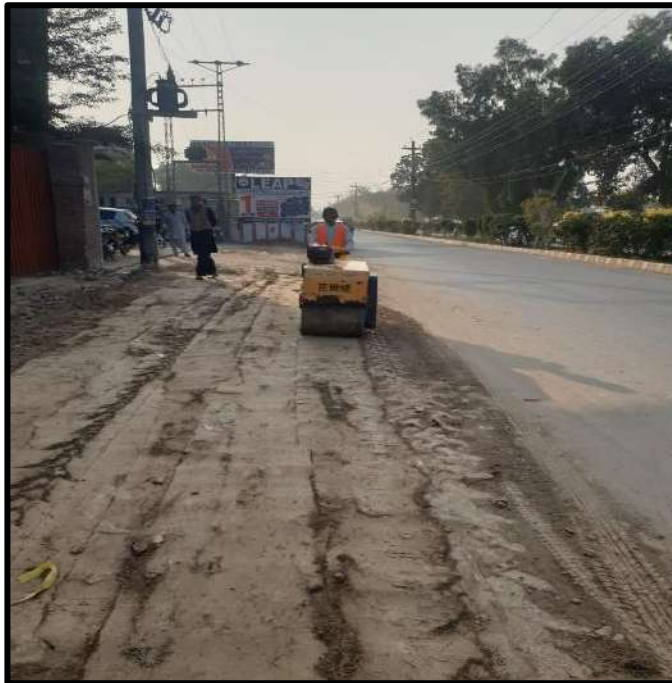
Picture 21: Restoration Work is in Progress
