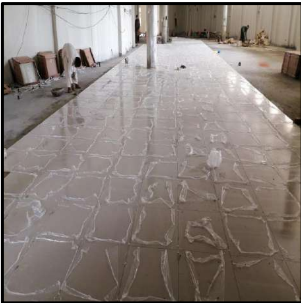
Picture 13: Museum Floor Work at Gulshan-e-Iqbal Park
