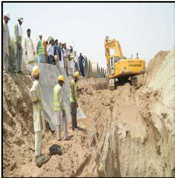
Picture 41: Levelling of Sewer Pipe is in Progress
