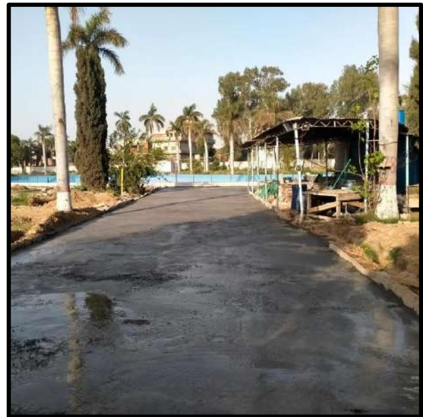
Picture 14: PCC for laying cobble Stone GI Park
